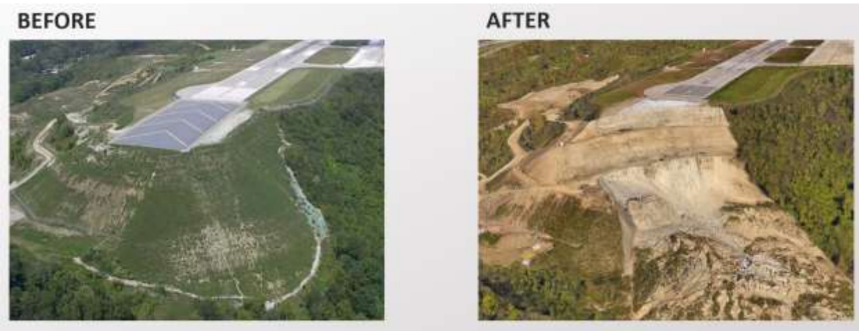
The Runway Safety Area on Runway 5 before and after the collapse
