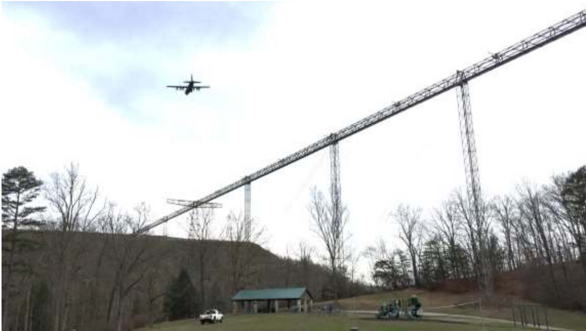
A West Virginia Air Guard C-130 flies over the approach lighting tower that spans approximately 3,000 feet in length
